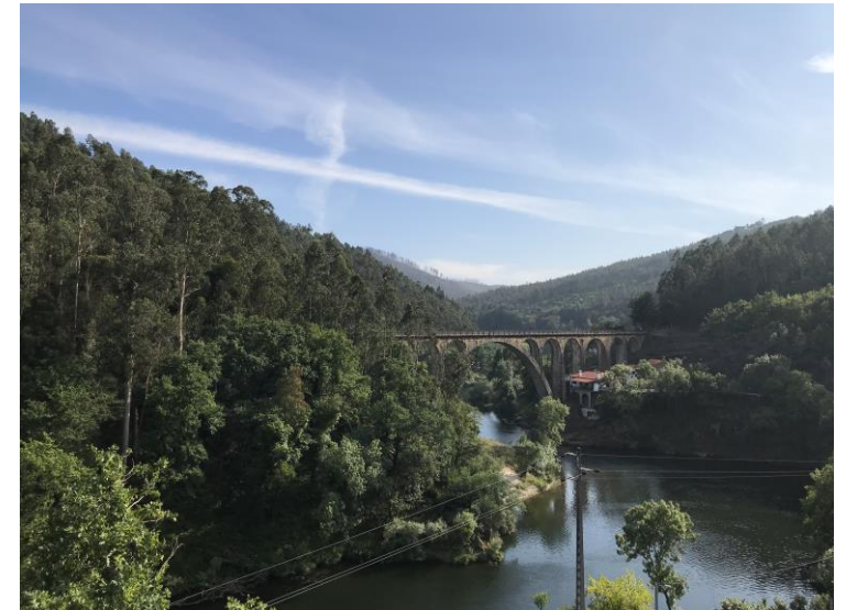
Source: TIS, Ecovia do Vouga - Sustainable Transport and Mobility Plan for Aveiro Region
